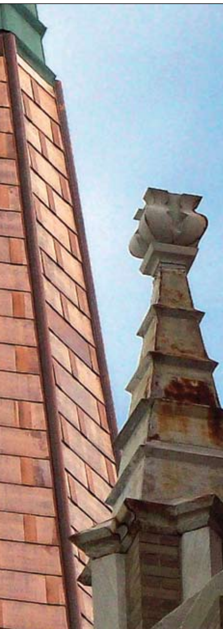
Copper shingles replace aluminum on the spires.
