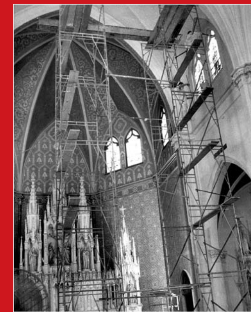
Scaffolding during the 1973 renovation.
