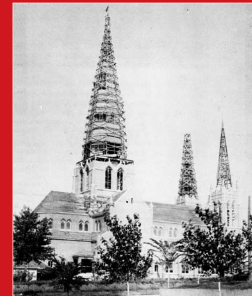
Original construction on Holy Family's spires, ca. 1914
